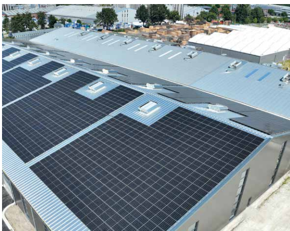
New hall at the Industrial location in Haren/Germany: photovoltaic system with an output of one megawatt peak.
