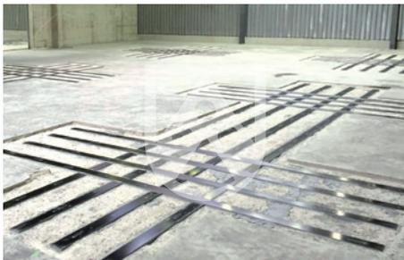
The supporting structure reinforcement made of carbon fibre reinforced composites increases the loadbearing safety
